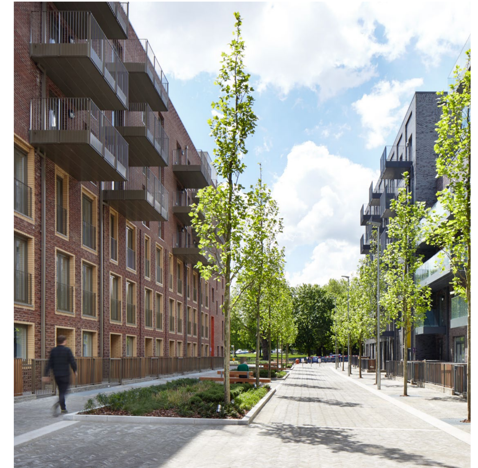
Burridge Gardens (Phase 1), Wandsworth
