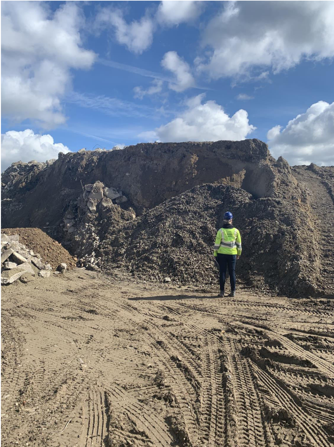
Photo 2: Waste piles already on 2m high waste platform, approximately 5m in height.
