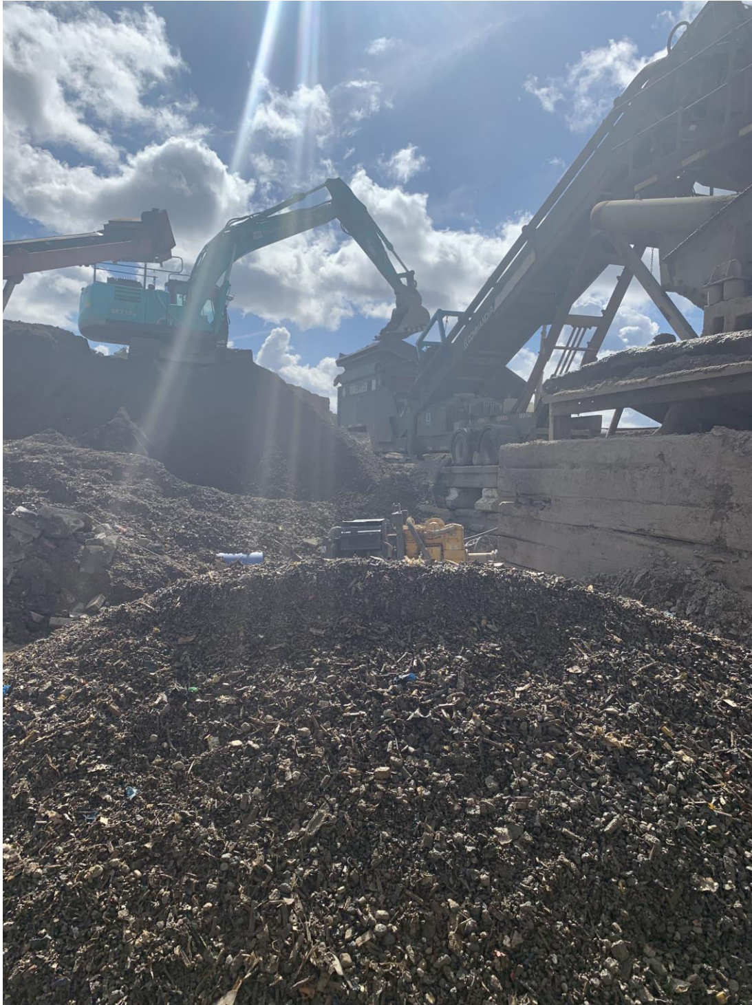
Photo 3: 360 Grabber operations being undertaken at height. Approximately 3m from plant base.
