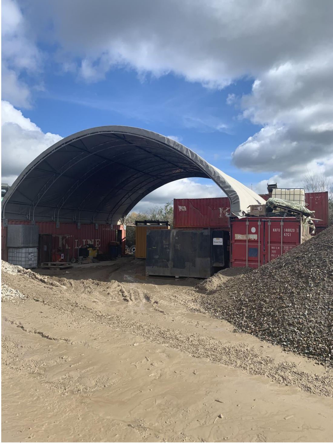
Photo 1: Gap in boundary behind hanger style storage unit.
