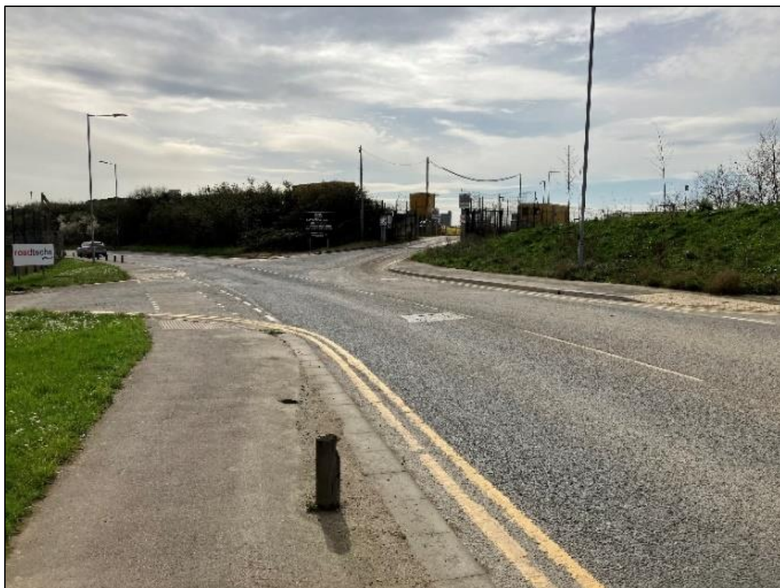
Photograph 5: Footways on Ferry Lane
