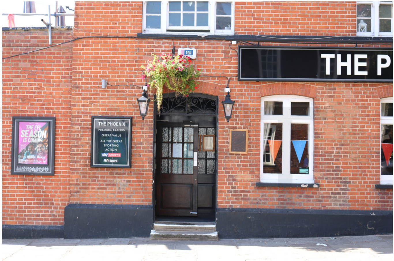
Surface-mounted services & conduit detract from façades
