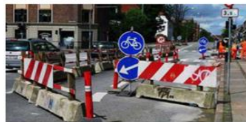
Cycling during road works
